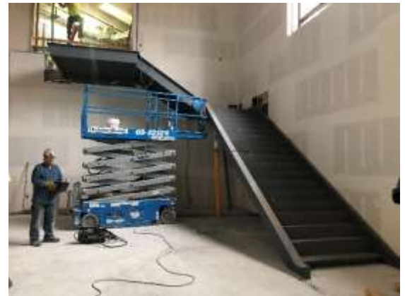
The steel for the grand stair installation is complete!
