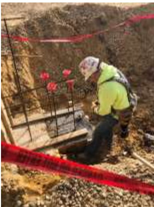
The photo on the left depicts the rebar framing and concrete work required for the canopy signage. The photo on the right is the masons installing the final brick.
