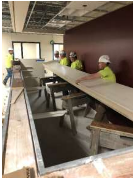
These three photos are various areas in the lower level Clinic / Med Surge Addition. Millwork installation is in full swing and when required, multiple man crews are needed to set long nurse station countertops (depicted in the middle photo).
