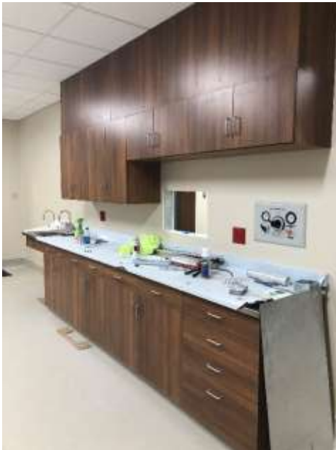
The millwork and flooring within CS have been installed! This is a view of the millwork in Process.
