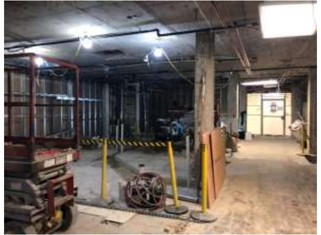
The exterior walls are framed up in the new Outpatient Clinic! Next step is to pour the concrete for the underground plumbing and frame the interior.
