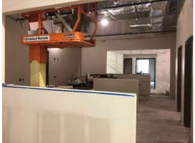
A view of the main nurse station in the upper level Clinic / Med Surge Addition. The walls have been taped and are ready for paint. Also seen is above ceiling rough in work taking place.
