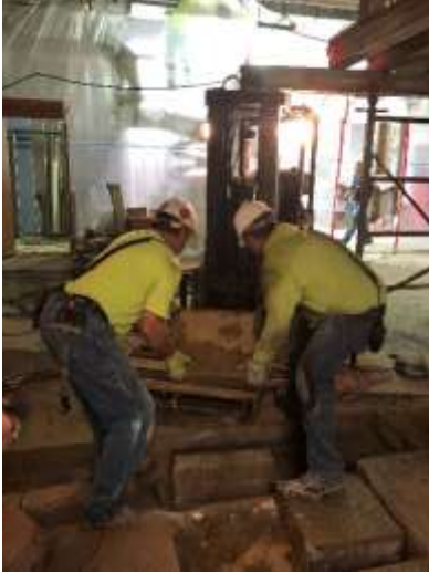
Teamwork makes the dream work! The Findorff crews work together to remove the existing beam in the new Outpatient Clinic.
