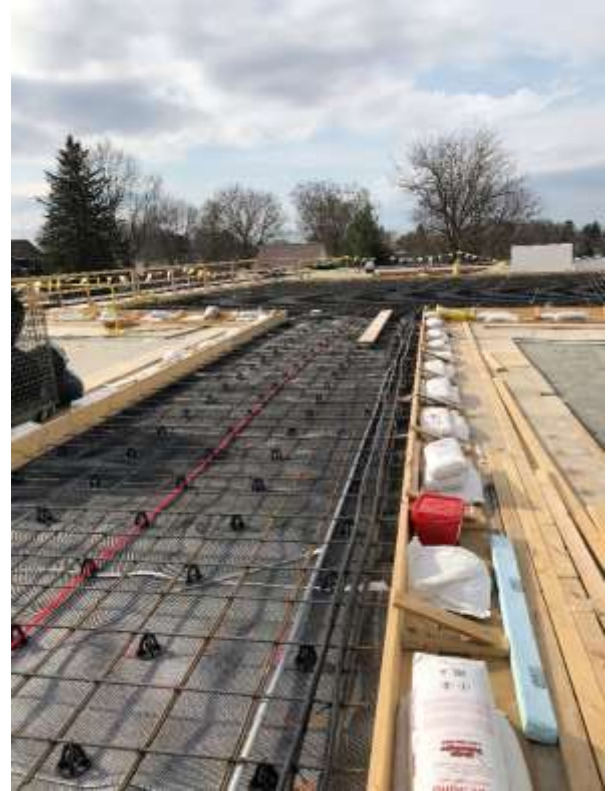
The rebar for the helipad has been installed and the snow melt system is well on its way. The snow melt system is the gray tubes seen on the right near the framing.
