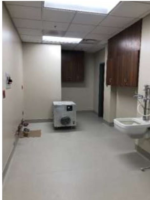
A view of the nearly completed Decontam room in CS.
