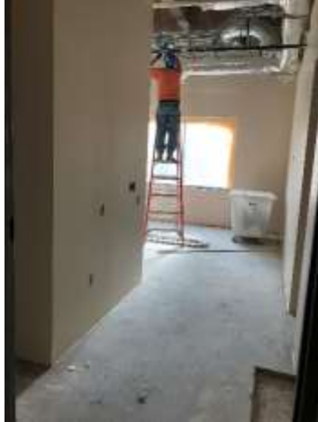
A corridor view (left) and patient room view (right) within the upper level Clinic / Med Surge Addition. Taping is finishing up and painting within the rooms has begun.
